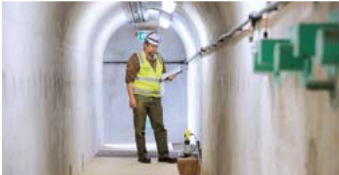
^ AN INSPECTION GALLERY INSIDE WARRAGAMBA DAM
