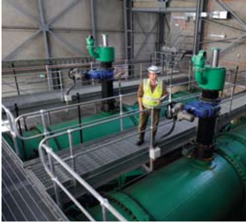
^ THE VALVE HOUSE, WARRAGAMBA
