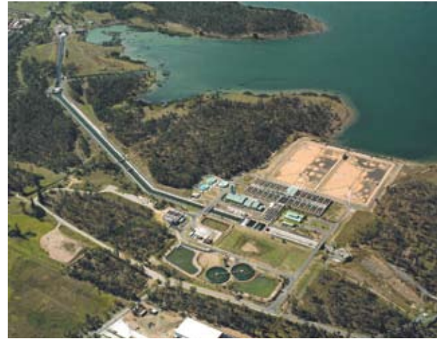
> AERIAL VIEW OF PROSPECT RESERVOIR
